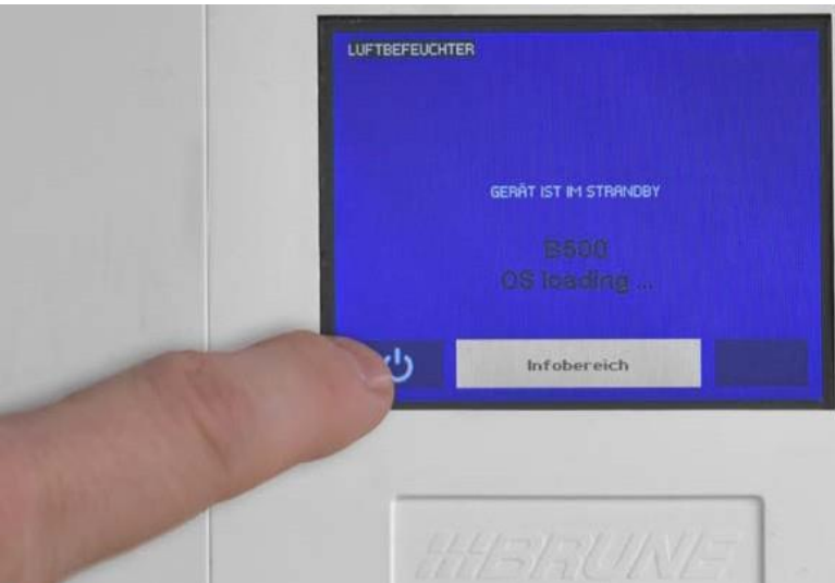
Fig. 4.3.6: Switching on the humidifier
